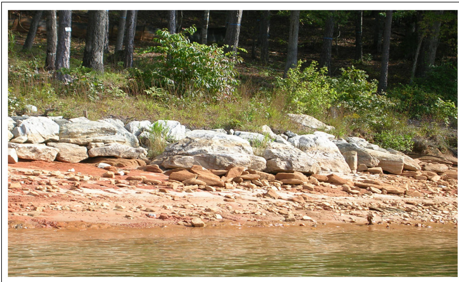
Figure 23. Enhanced Riprap (with Boulders and Plantings)
